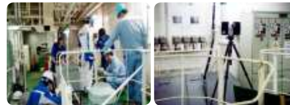
Pump piping line check
